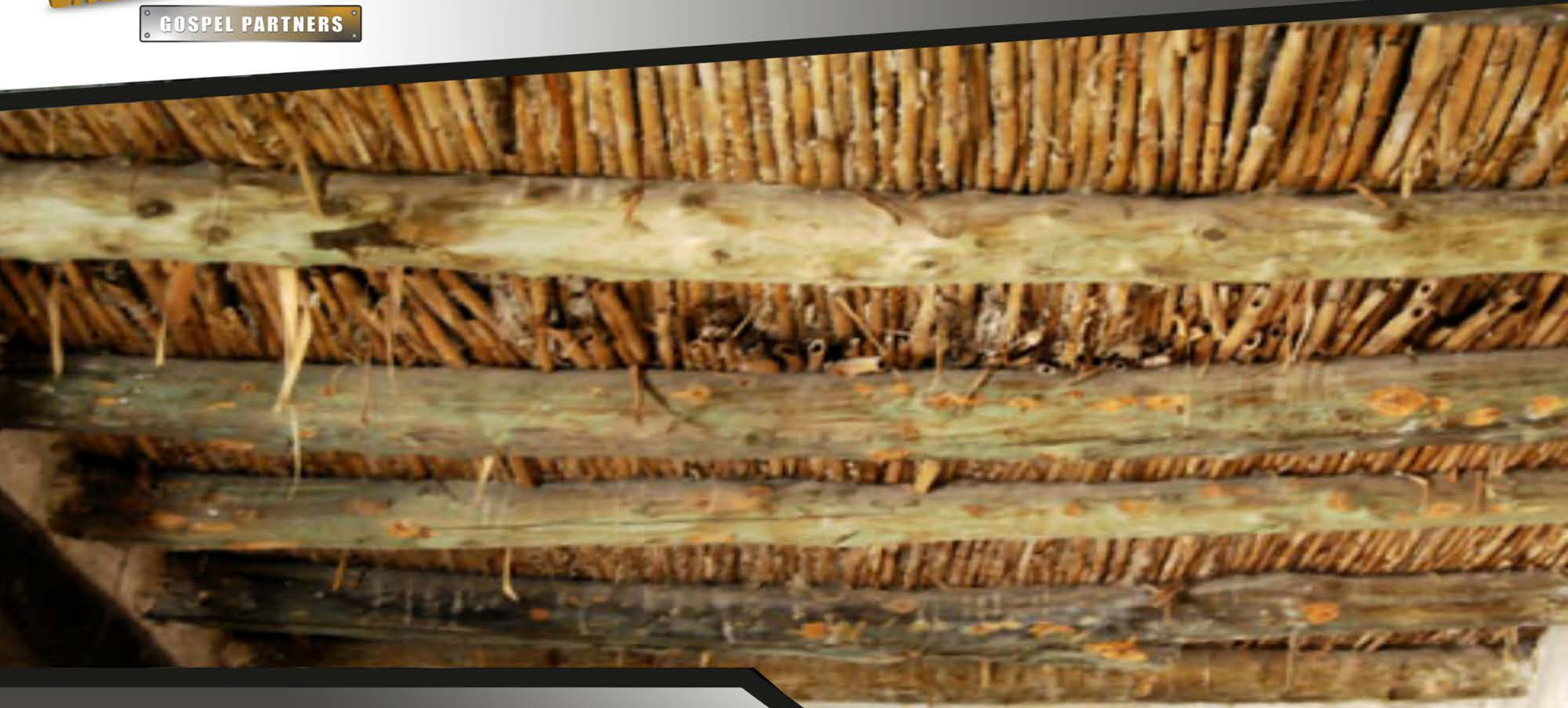
Ceiling of roof made of timber and reeds
